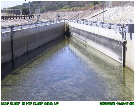
Figure 1.12. Fish Screens and Cleaning Brushes in Robles Canal.
