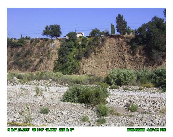
Figure 4.15. East Bank of Ventura River Located at RM 9.6 Showing Some Recent Bank Failure,
