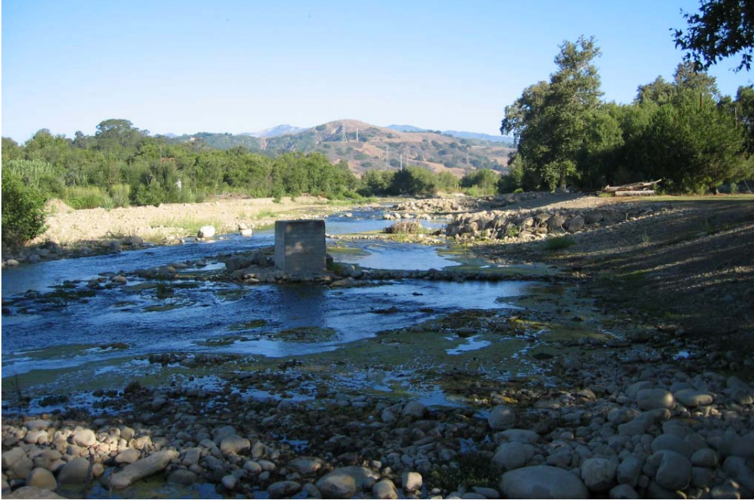
Figure 10. Picture Downstream of Proposed Well Locations Looking Upstream. Groins are Seen Along the Left Bank. The Concrete Structure is an Existing Well Operated by City of Ventura.
